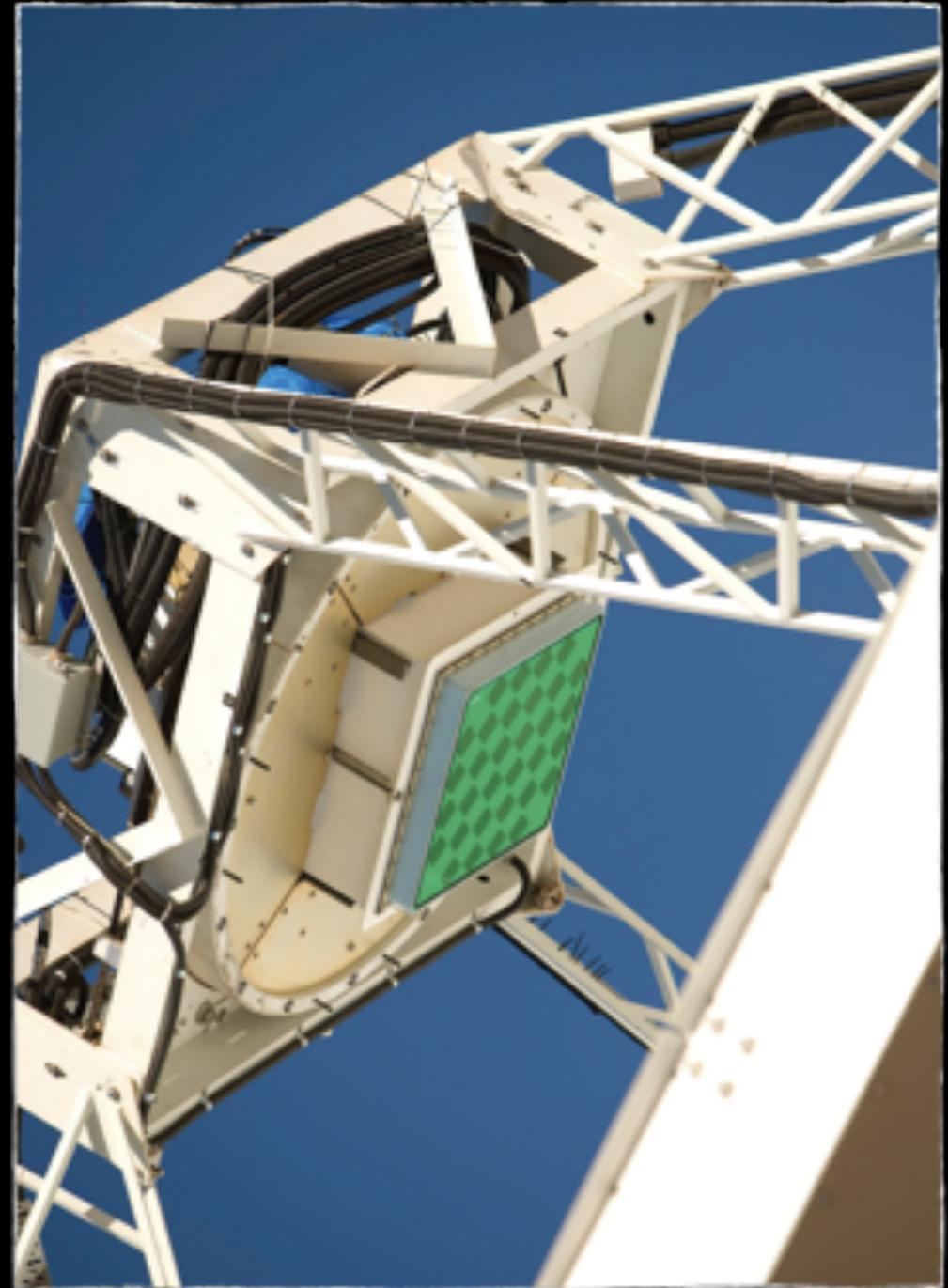
Chequer board sensor array on each dish
